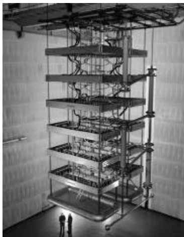
Fig. 6: Quadruple valve tower (photograph taken in the high-voltage test field of the University of Karlsruhe / Germany).
